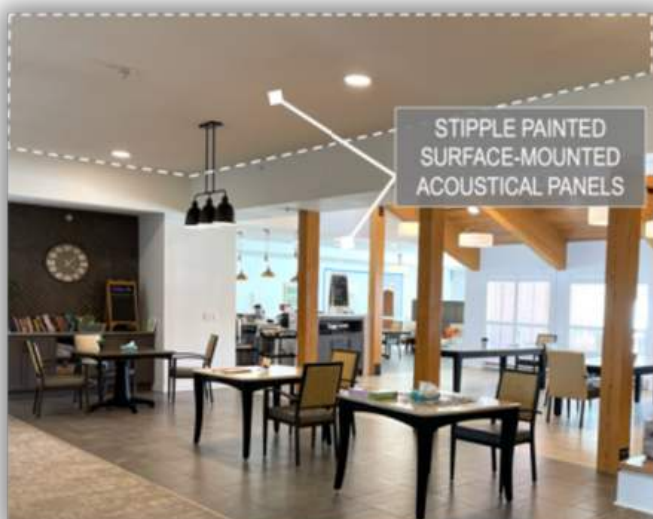
Stipple-painted, surface-mounted acoustical panels give the smooth look of gypsum board.
